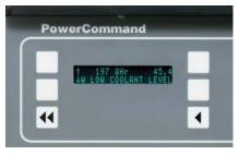
The PowerCommand control is provided with an alphanumeric display capable of displaying 2 lines of data with approximately 20 characters per line. The display is accompanied by a set of six tactile-feel membrane switches that are used by the operator to navigate through
