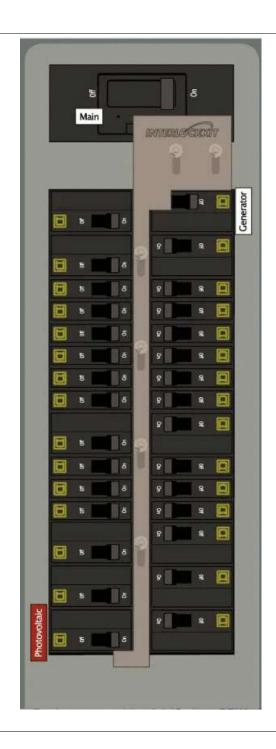
This Interlock Kit mounts to SQUARE D electrical panels with the following features:
