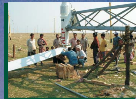
Installing Blades in West Bengal, India
